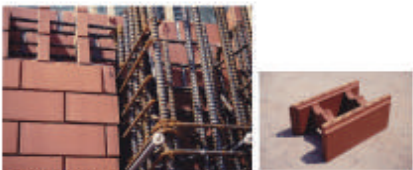
補強組立構造 (Reinforced Masonry)
